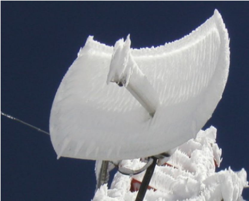
Figure ATL 17: Effect of ice on a parabolic grid antenna
