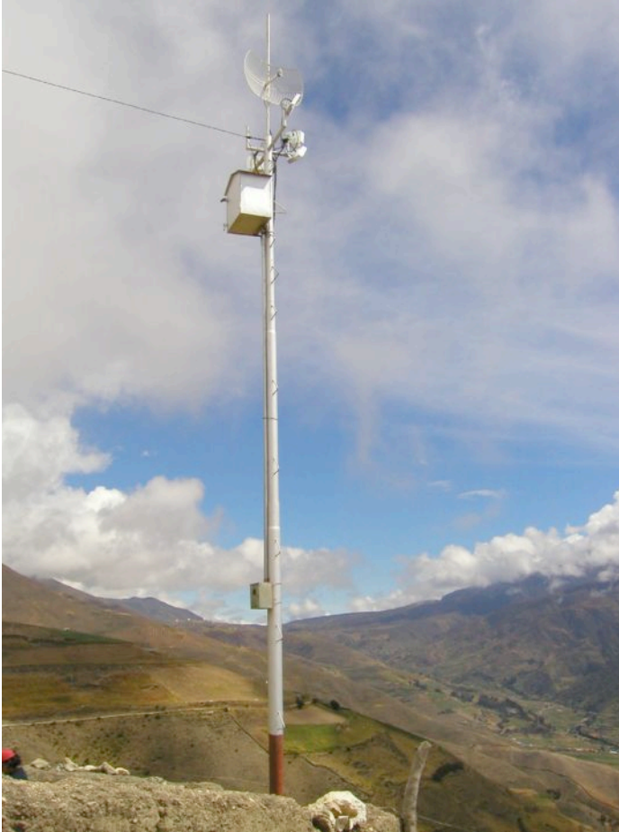
Figure 7.3: A simple self-supporting tower.
